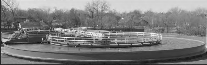
Wastewater Treatment Solutions
