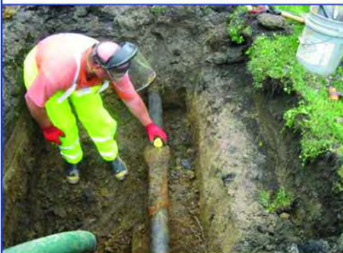
Splash in the Trenches
